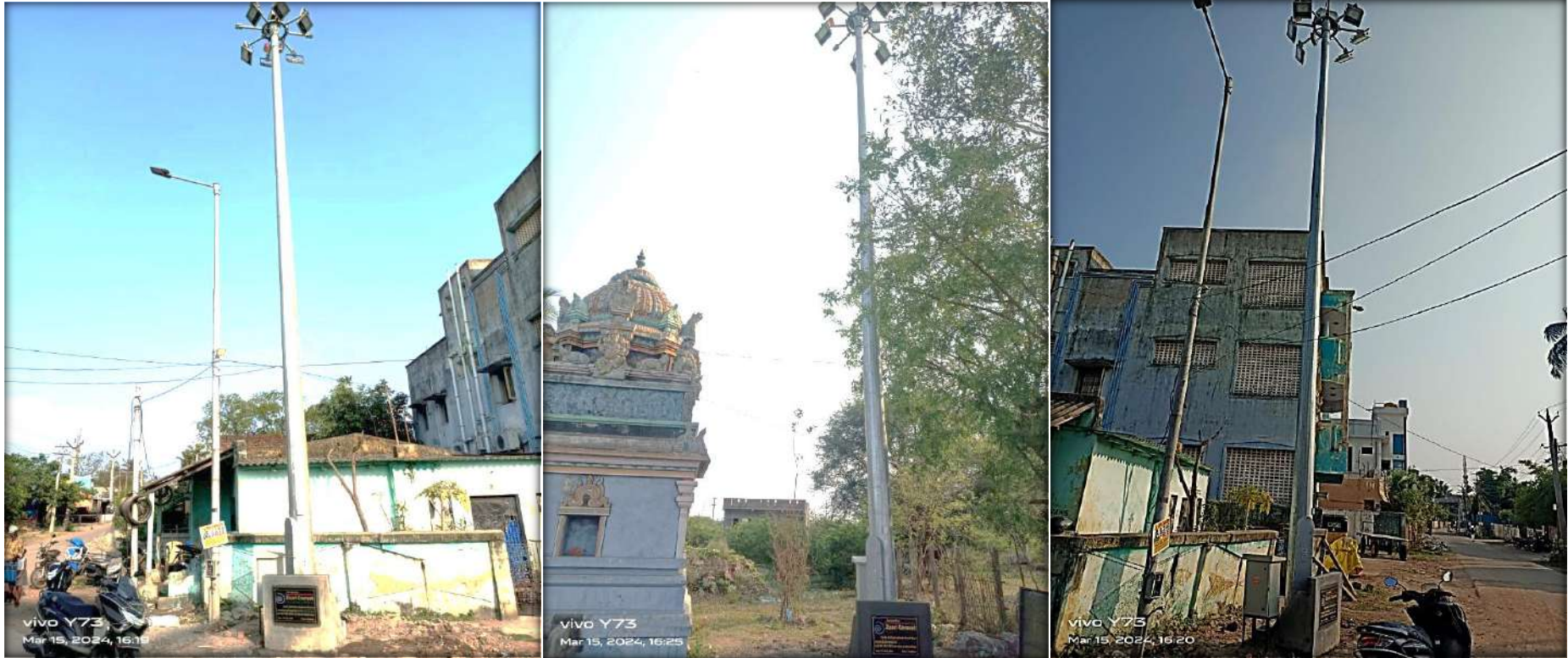
High mast lights
