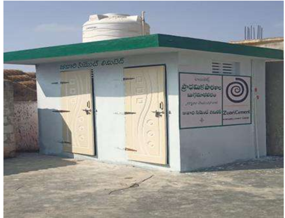
Toilet Construction at Buggamadavaram Primary School
