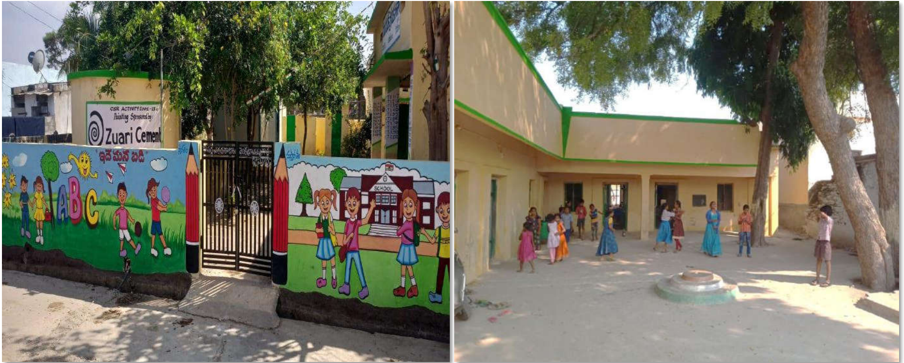
Renovation and Wall Paintings at Govt School
